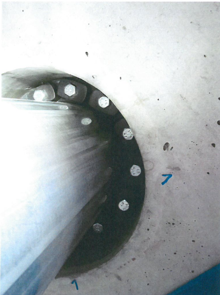
Figure 3: The link chain seal installed for sealing the annular gap
